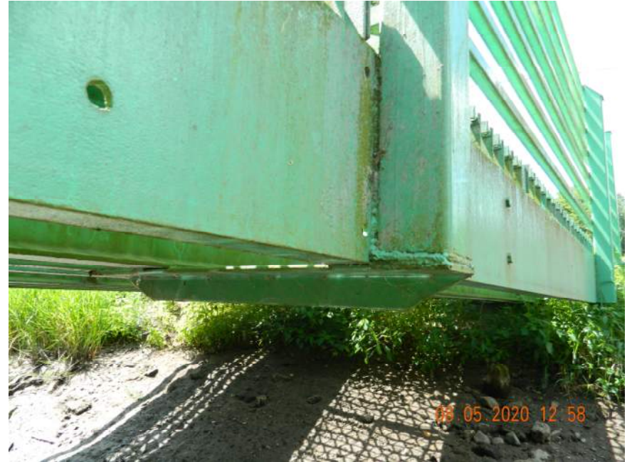
TYP. CONNECTION OF RAIL TO BEAMS
