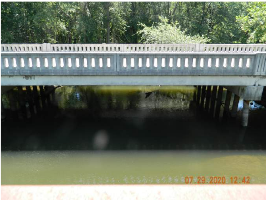
CHANNEL UPSTREAM LOOKING SOUTH
