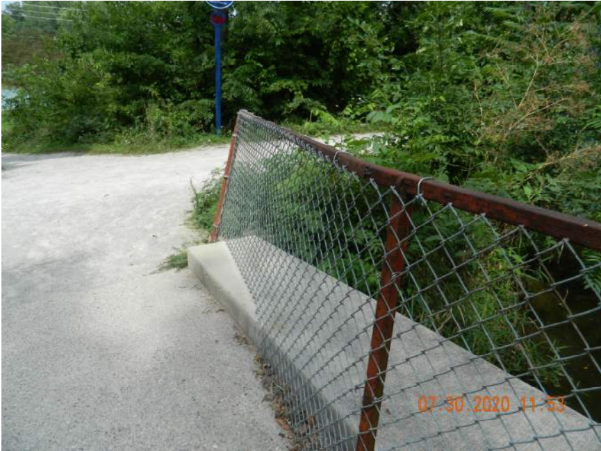
NORTH RAIL BENT AT WEST END
