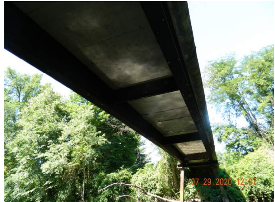
UNDERSIDE OF MAIN SPAN
