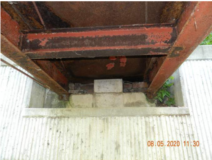
BEARINGS AT EAST END
