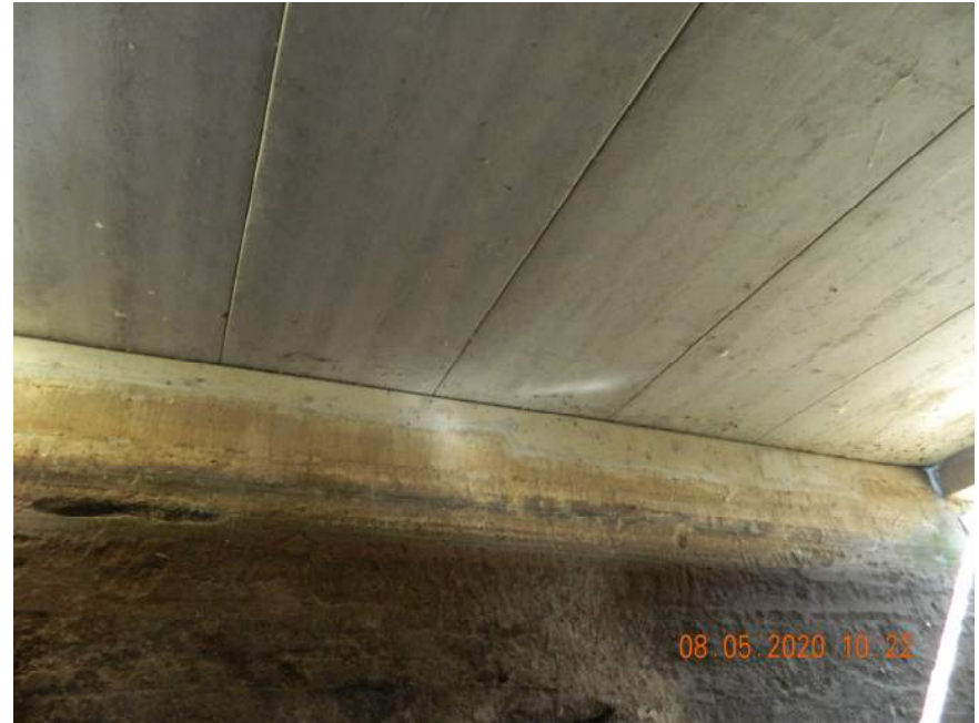
TYPICAL UNDERSIDE OF NORTH SPAN
