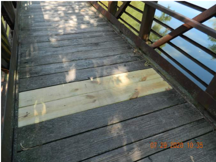
REPLACED TIMBER BOARDS NEAR MIDSPAN
