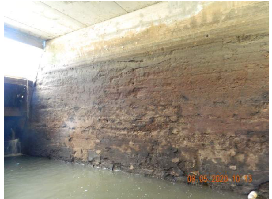
CENTER PIER, SOUTH FACE
