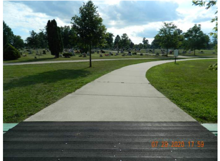
APPROACH LOOKING WEST
