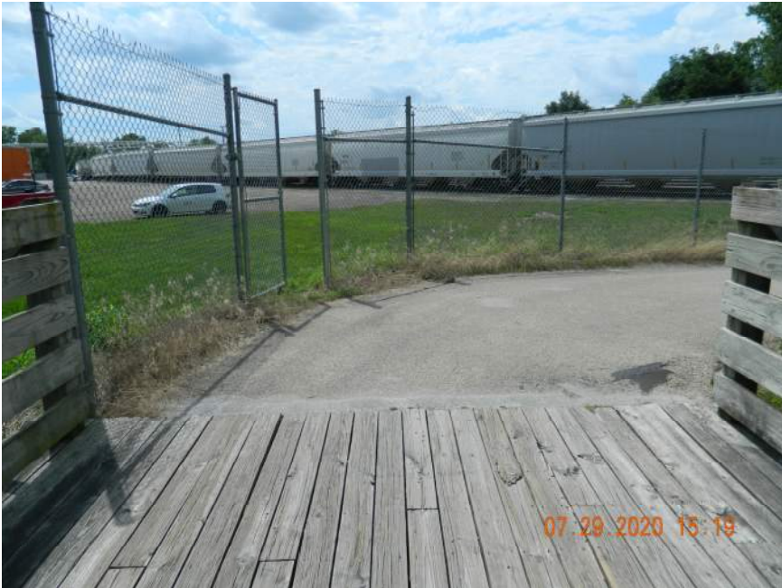
APPROACH LOOKING WEST
