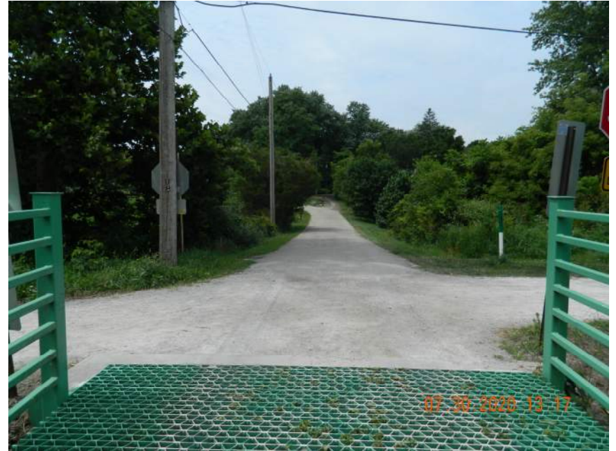
APPROACH LOOKING WEST
