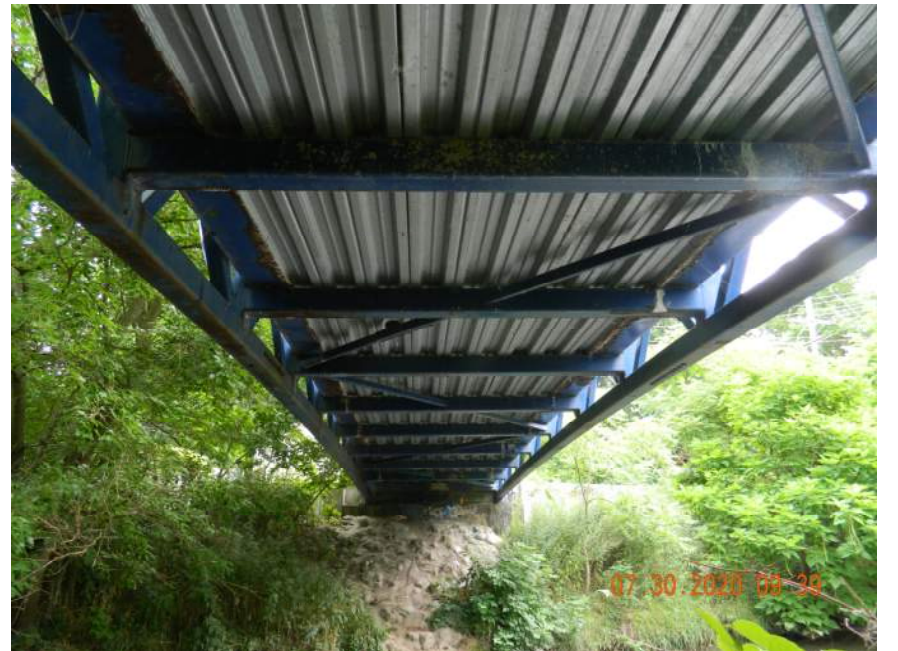
UNDERSIDE OF BRIDGE LOOKING NORTH
