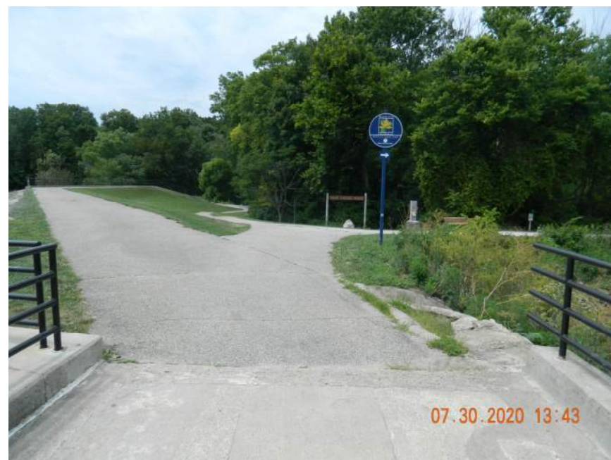
APPROACH LOOKING WEST
