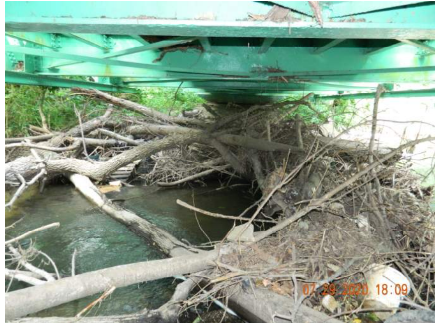
DEBRIS UNDER BRIDGE AND BETWEEN LATERALS
