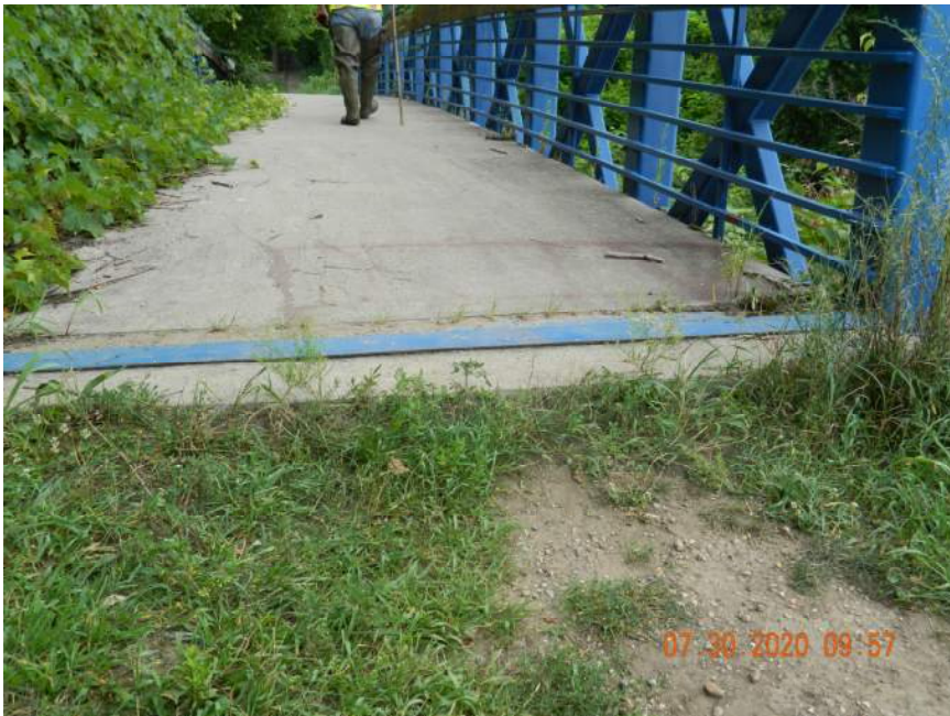
NO APPROACH AND DROP OFF AT SOUTH APPROACH
