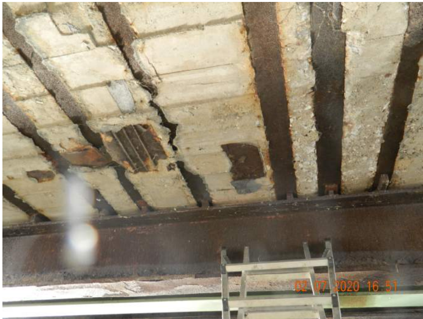
UNDERSIDE OF EAST SPAN
