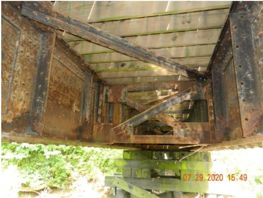
TYPICAL UNDERSIDE OF MAIN SPAN
