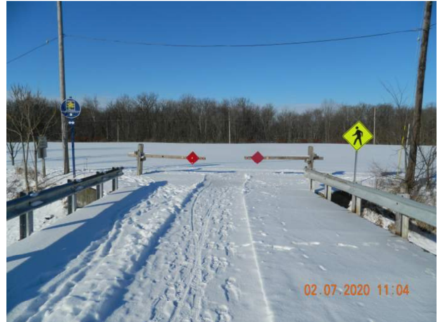
APPROACH LOOKING WEST
