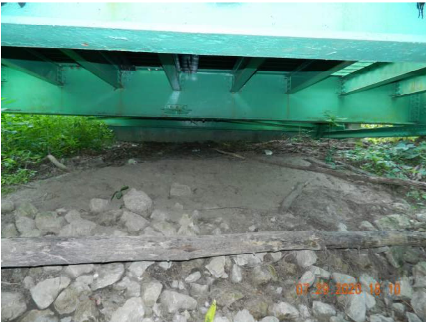
DISPLACED RIPRAP AT WEST SPILLSLOPE
