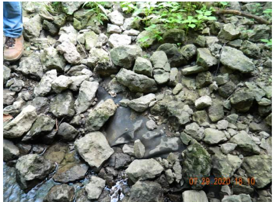
EXPOSED GEOTEXTILES AT WEST SPILL SLOPE
