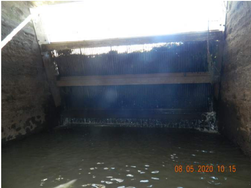
CANAL SCREEN AT SOUTH SPAN
