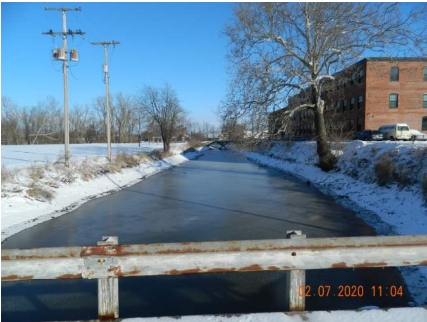
DOWNSTREAM CHANNEL LOOKING NORTH
