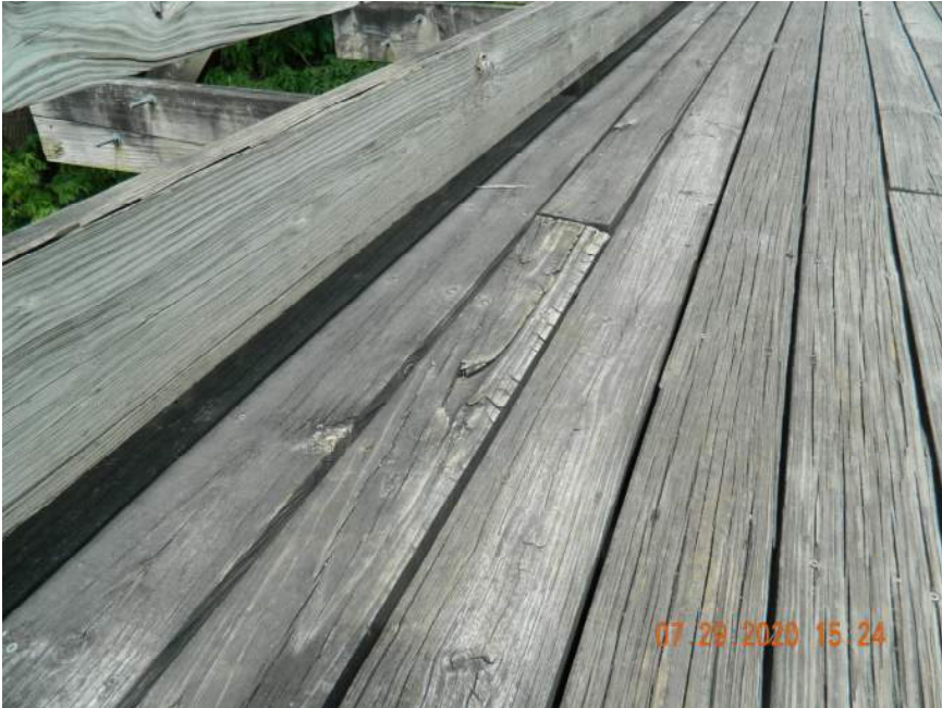
CHECKING OF TIMBER DECK
