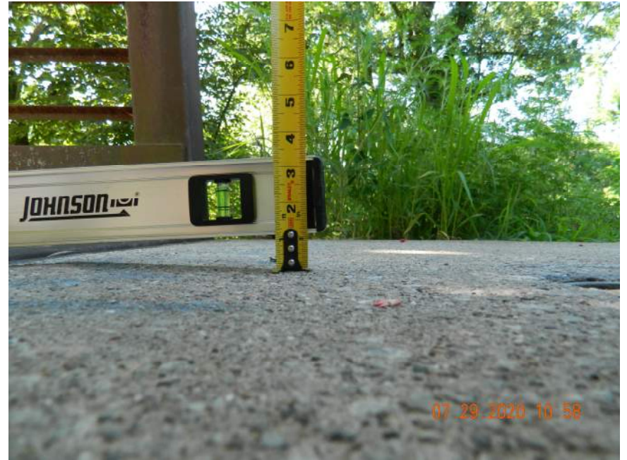
WEST APPROACH END WITH 1" VERTICAL OFFSET
