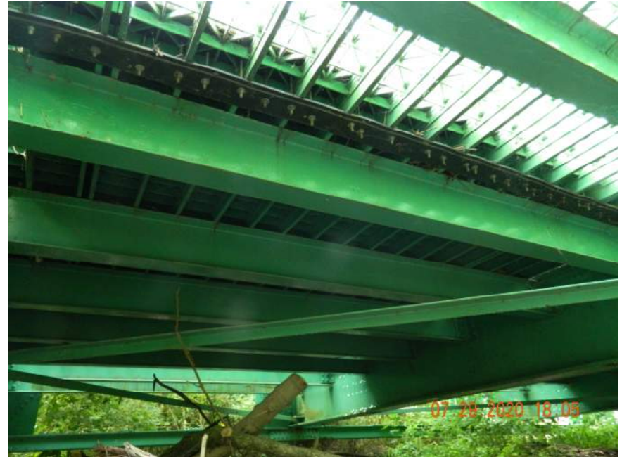
TYPICAL UNDERSIDE OF BRIDGE
