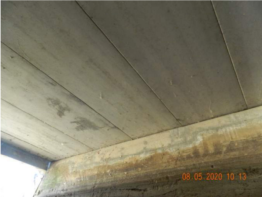
UNDERSIDE OF SOUTH SPAN
