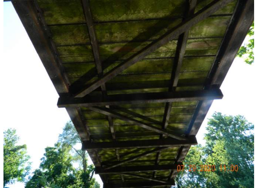
TYPICAL UNDERSIDE OF STRUCTURE
