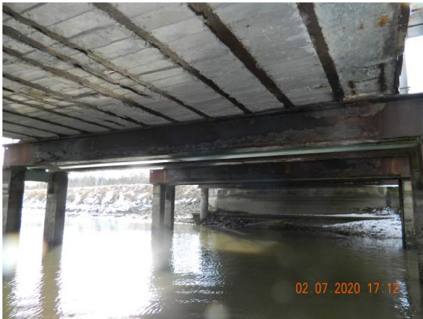
EAST BENT CAP BEAM AT BENT 4
