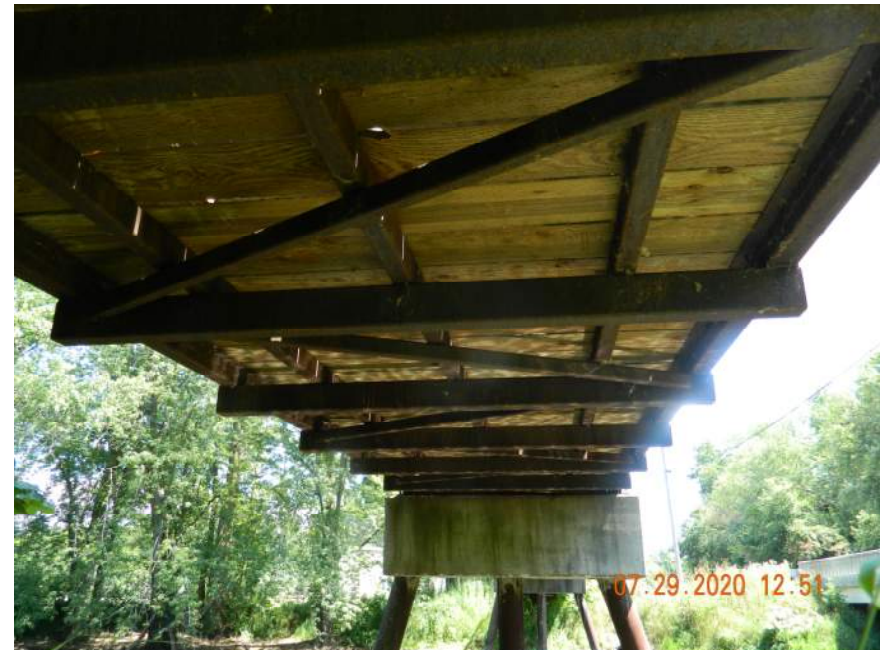
TYPICAL UNDERSIDE OF BRIDGE
