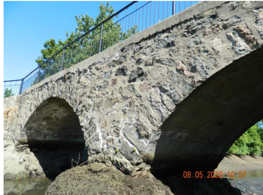
TYPICAL MASONRY CONDITION AT BRIDGE
