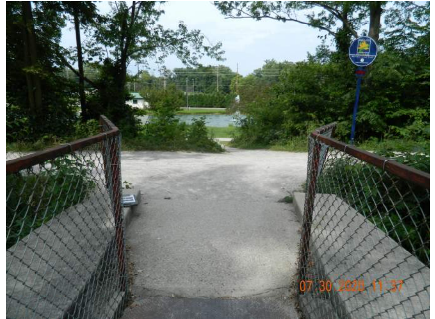
APPROACH LOOKING WEST
