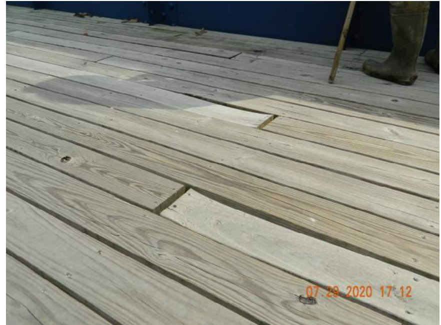
WARPING IN DECK TIMBER BOARDS
