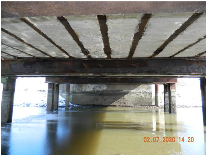
TYPICAL UNDERSIDE LOOKING EAST
