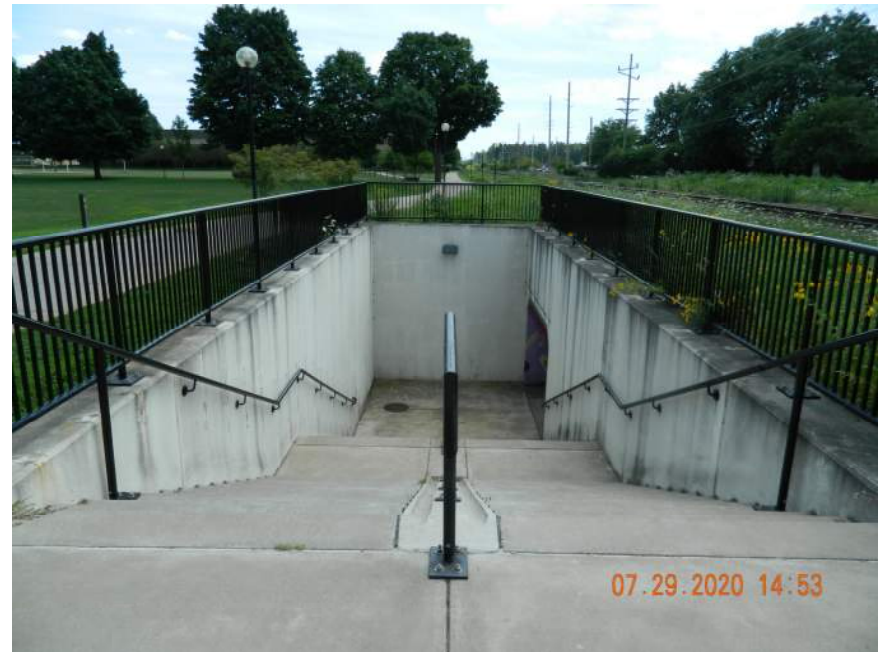
EAST STAIRS LOOKING SOUTH
