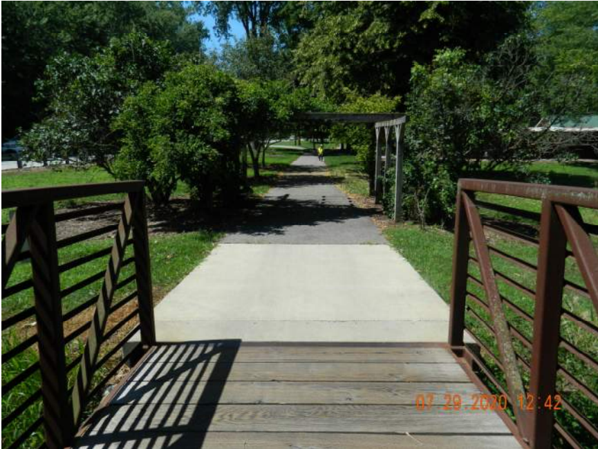
APPROACH LOOKING WEST
