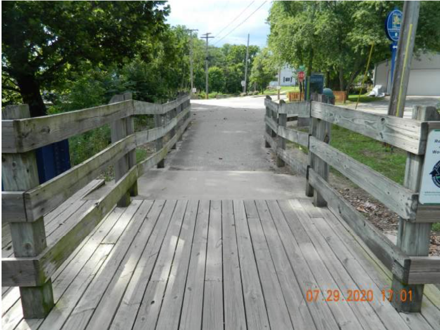
APPROACH LOOKING WEST
