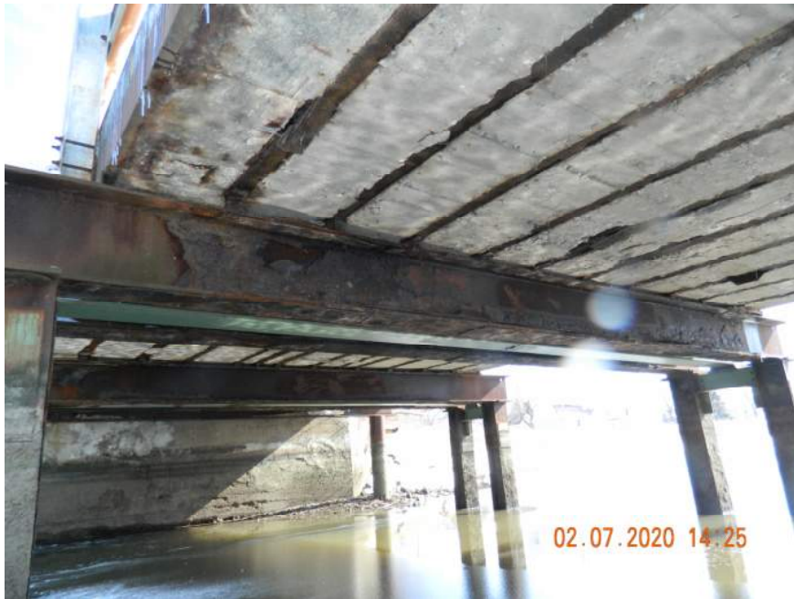
WEST BENT CAP BEAM AT BENT 4
