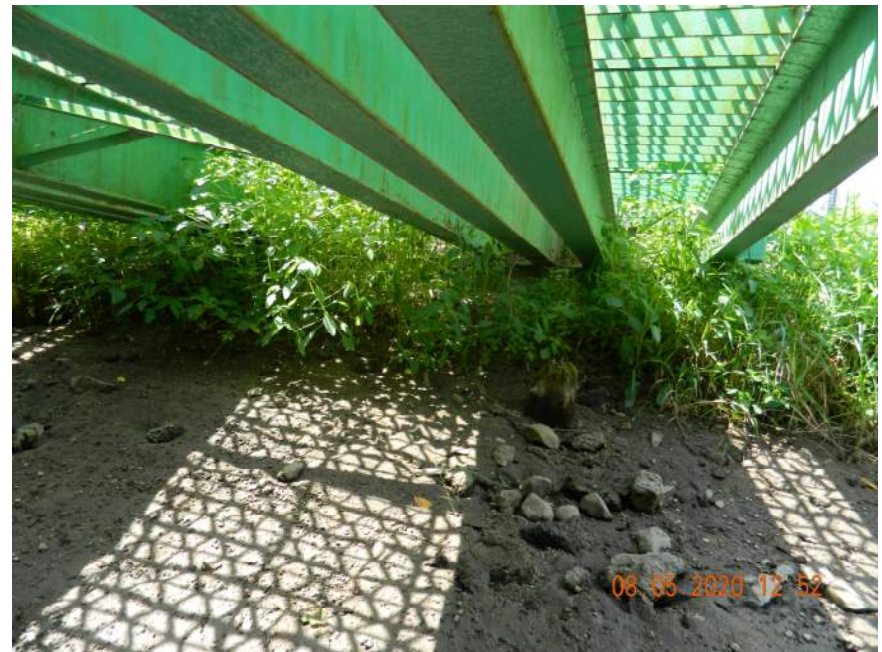
VEGETATION AT WEST END OF BRIDGE
