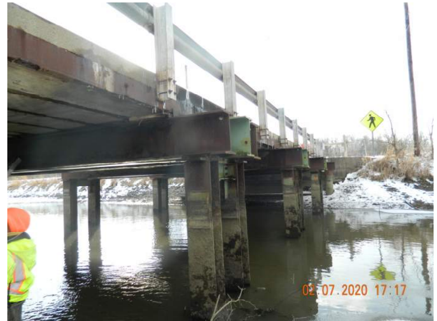
NORTH COPING, END OF BEAMS & PILES AT BENTS 3, 4 & 5
