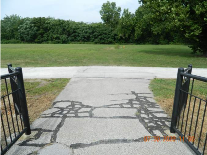
APPROACH LOOKING WEST
