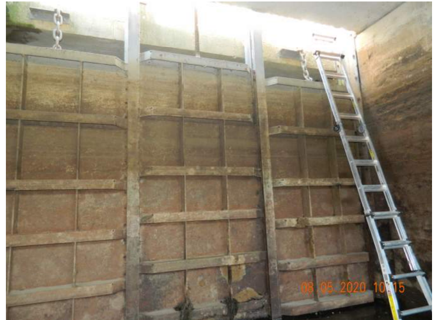
GATE AT SOUTH SPAN
