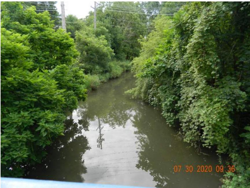
CHANNEL UPSTREAM LOOKING EAST
