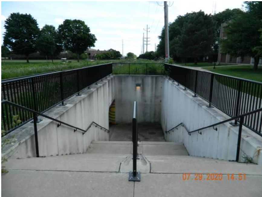
WEST STAIRS LOOKING SOUTH
