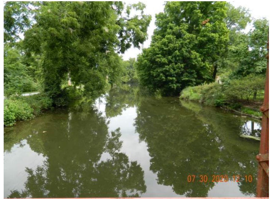
DOWNSTREAM CHANNEL LOOKING NORTH
