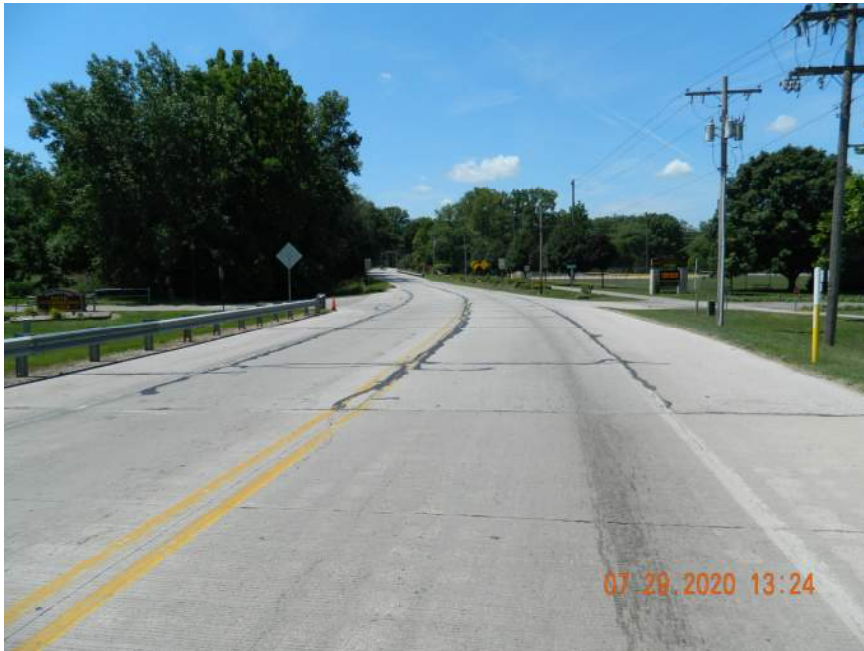
APPROACH LOOKING WEST
