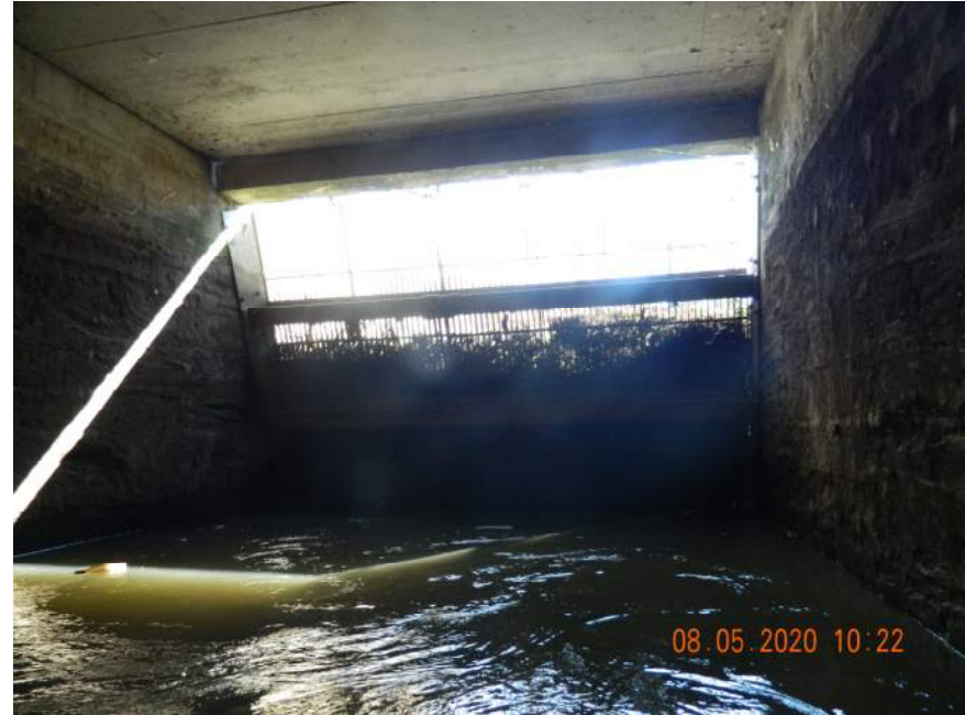
CANAL SCREEN AT NORTH SPAN
