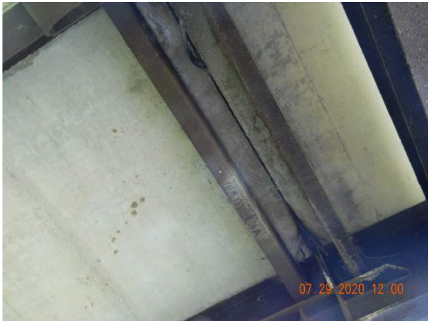
UNDERSIDE OF FAILED EAST EXPANSION JOINT DECK
