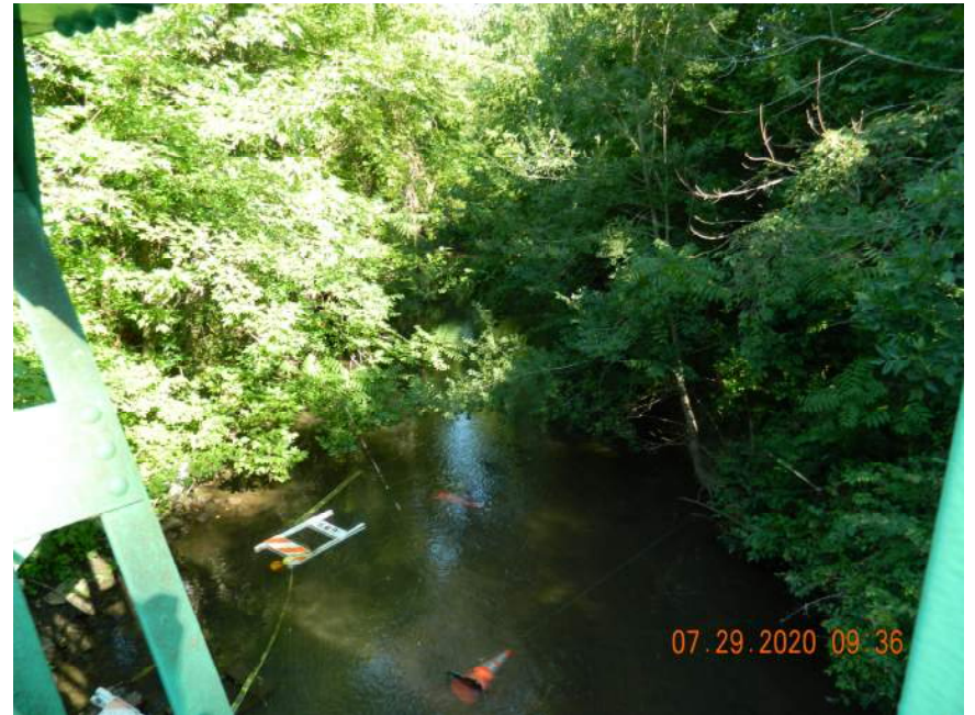
DOWNSTREAM CHANNEL LOOKING NORTH
