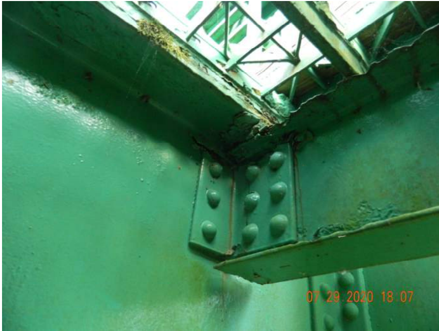
TYP. SECTION LOSS AT TOP FLANGE OF STRINGER/ FB CONN.
