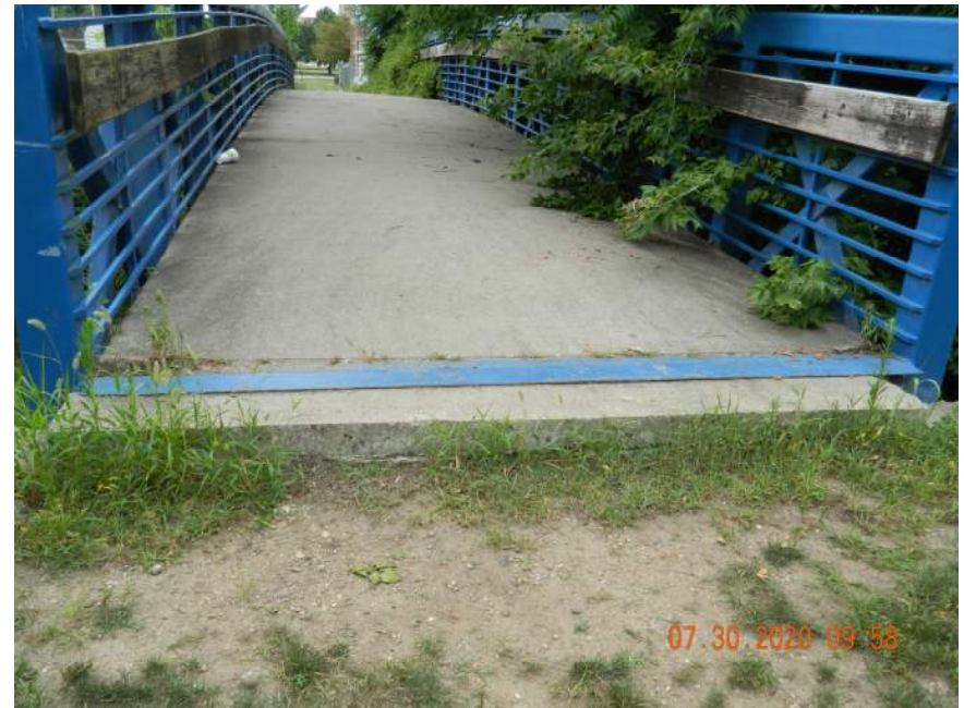
NO APPROACH AND DROP OFF AT NORTH APPROACH
