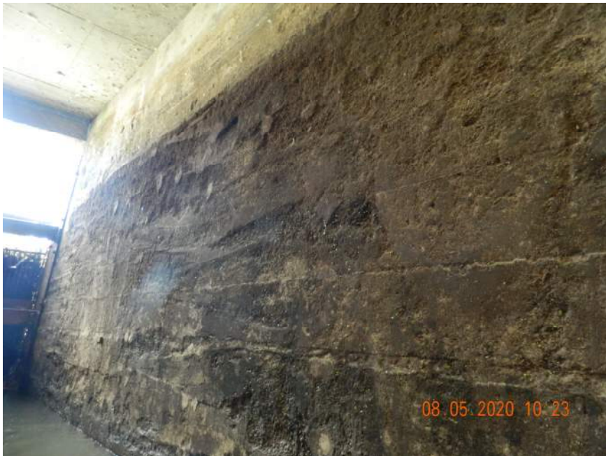
CENTER PIER, NORTH FACE
