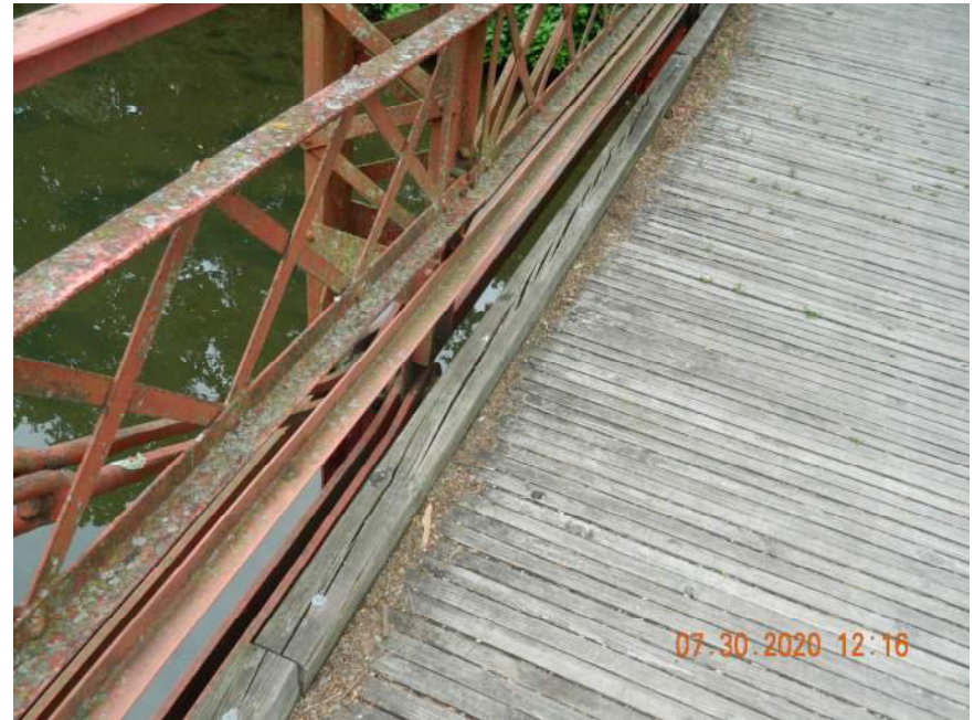
TYP. SPLITTING OF TIMBER CURBS
