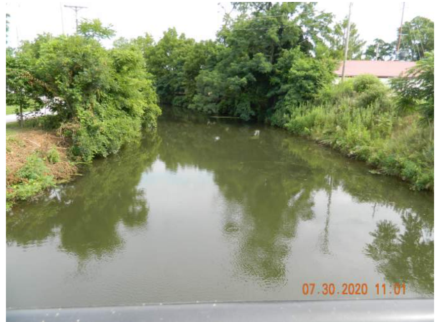
DOWNSTREAM CHANNEL LOOKING NORTH
