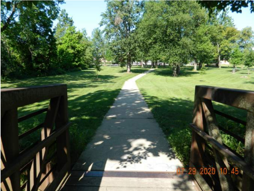
APPROACH LOOKING WEST
