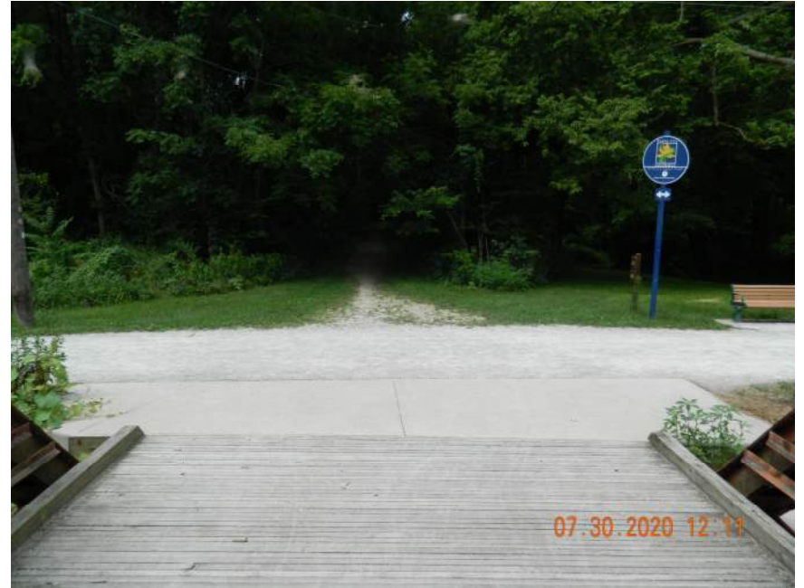
APPROACH LOOKING WEST
