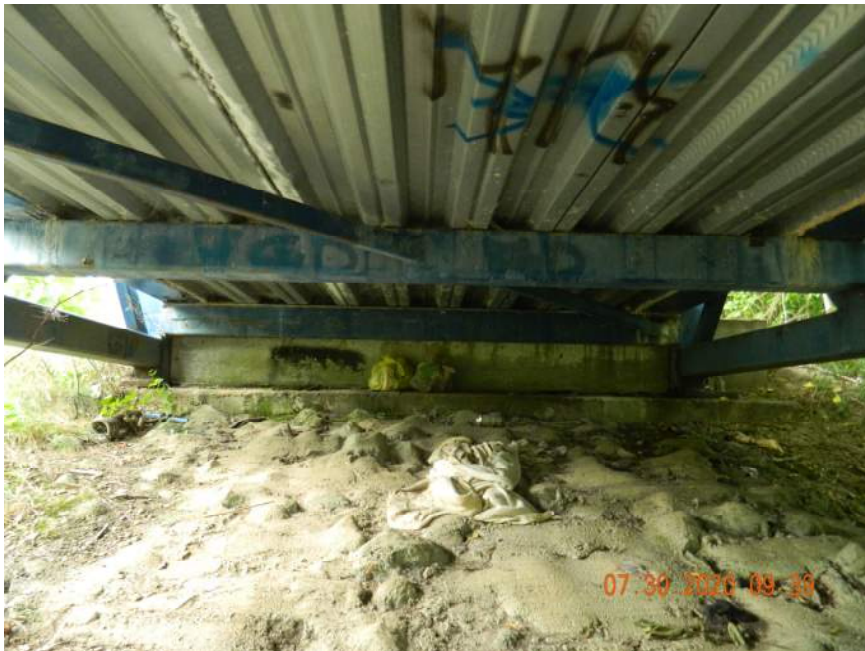
SOUTH END BENT
