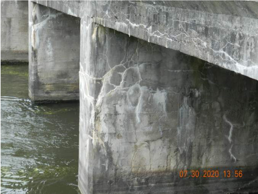
HEAVY CRACKING WITH LEACHING IN PIER WALLS
