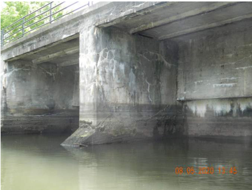
CRACKING AND SCALING IN WEST PIER
