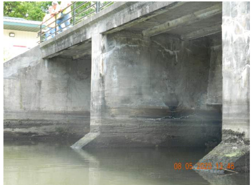
CRACKING AND SCALING IN EAST PIER
