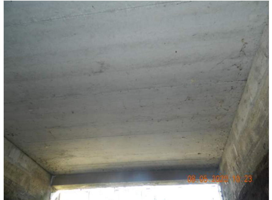
TYPICAL UNDERSIDE OF NORTH SPAN
