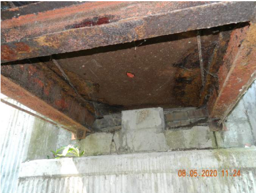
BEARINGS AT WEST END
