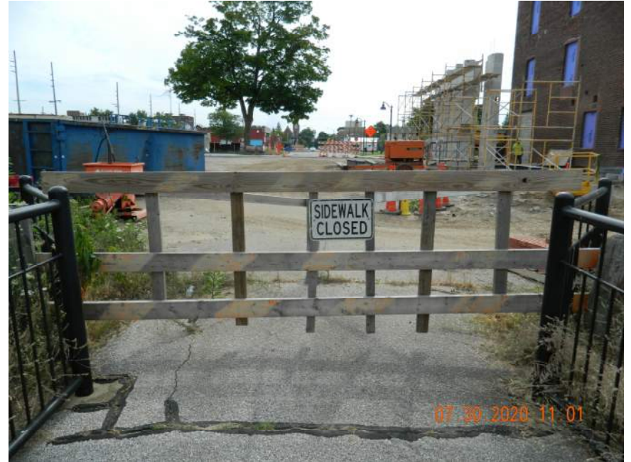
APPROACH LOOKING EAST (CLOSED DUE TO CONSTR.)
