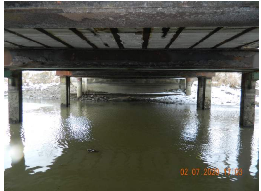
TYPICAL UNDERSIDE LOOKING WEST
