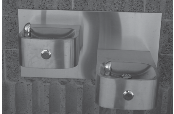
Fountains Connected to a Central Chiller
