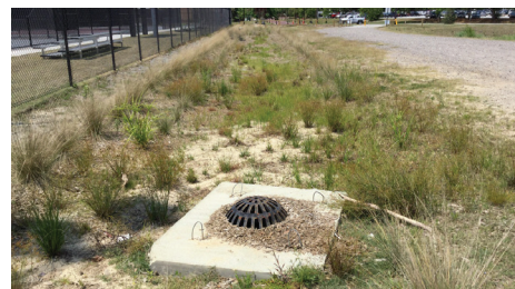
14 MULCH (NONE), 18 OUTLET DEBRIS, & 22 UNDESIRABLE VEGETATION (MARGINAL)
