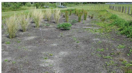
14 MULCH (<2"), 22 UNDESIRABLE VEGETATION (MARGINAL) & 24 PLANT DENSITY (MARGINAL)
